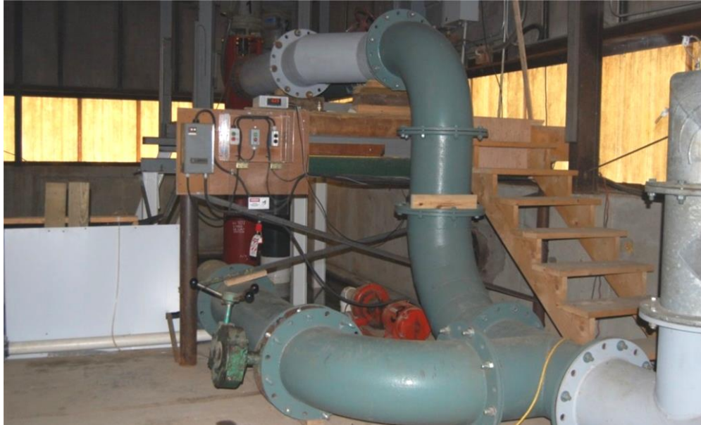
Figure 7: Photograph Showing Laboratory Pumps
