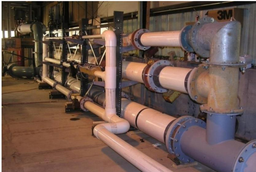
**Figure 4: Photograph Showing Laboratory Flow Meters**
