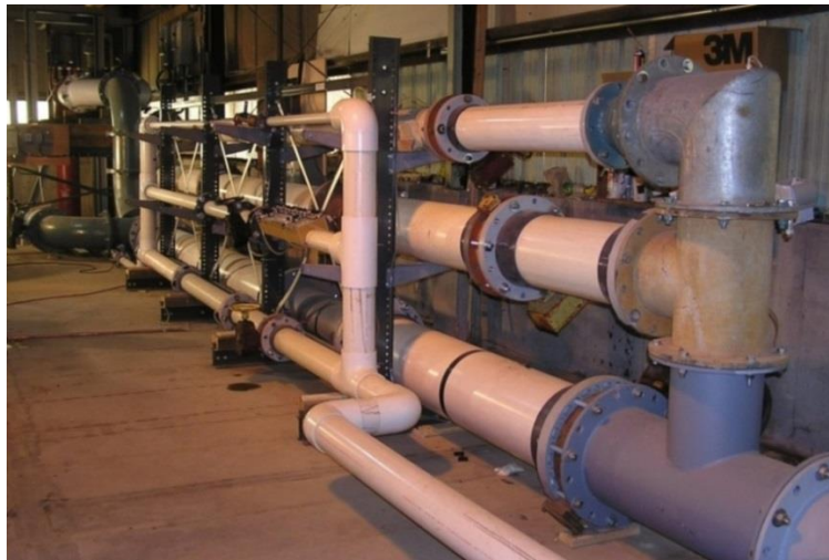
Figure 4: Photograph Showing Laboratory Flow Meters
